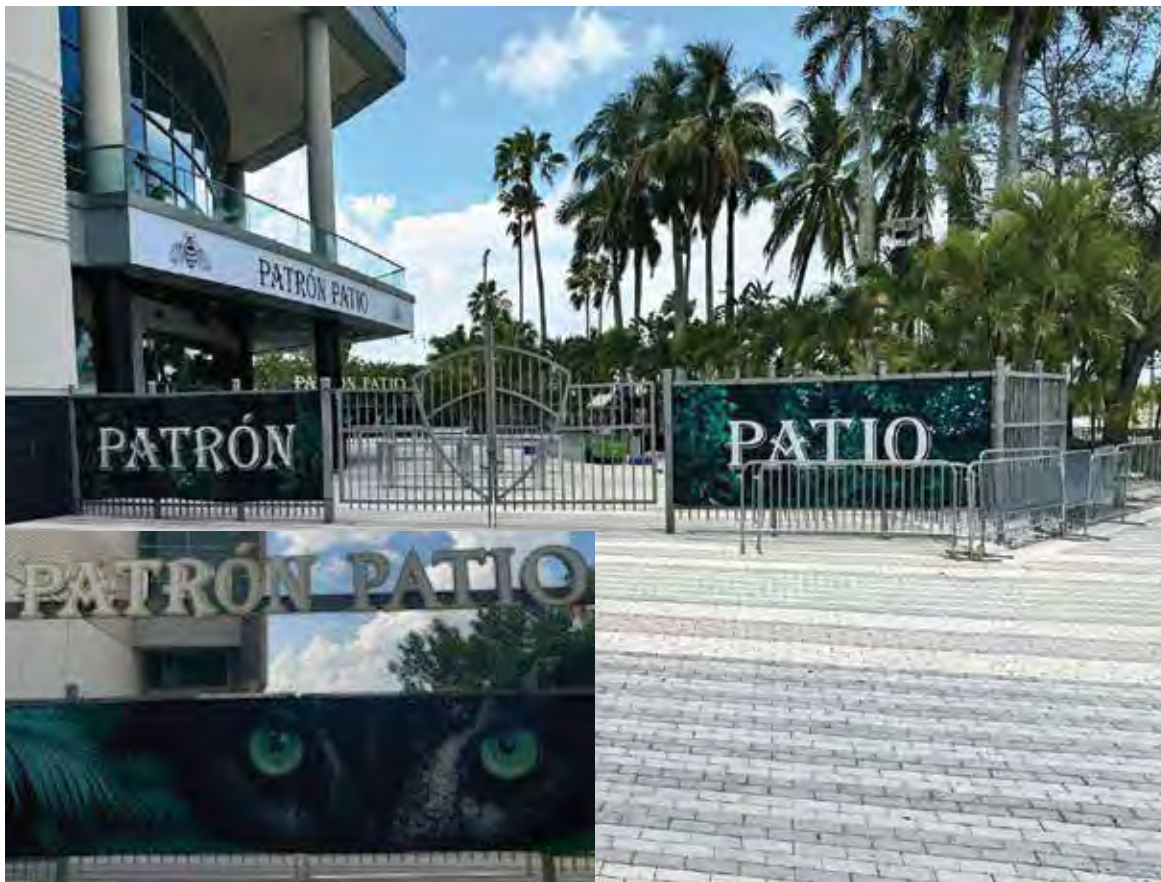
13 oz Baner material attached to (2) 4x4 Post with heavy duty Zipties Size: 52' FT x 5' FT
