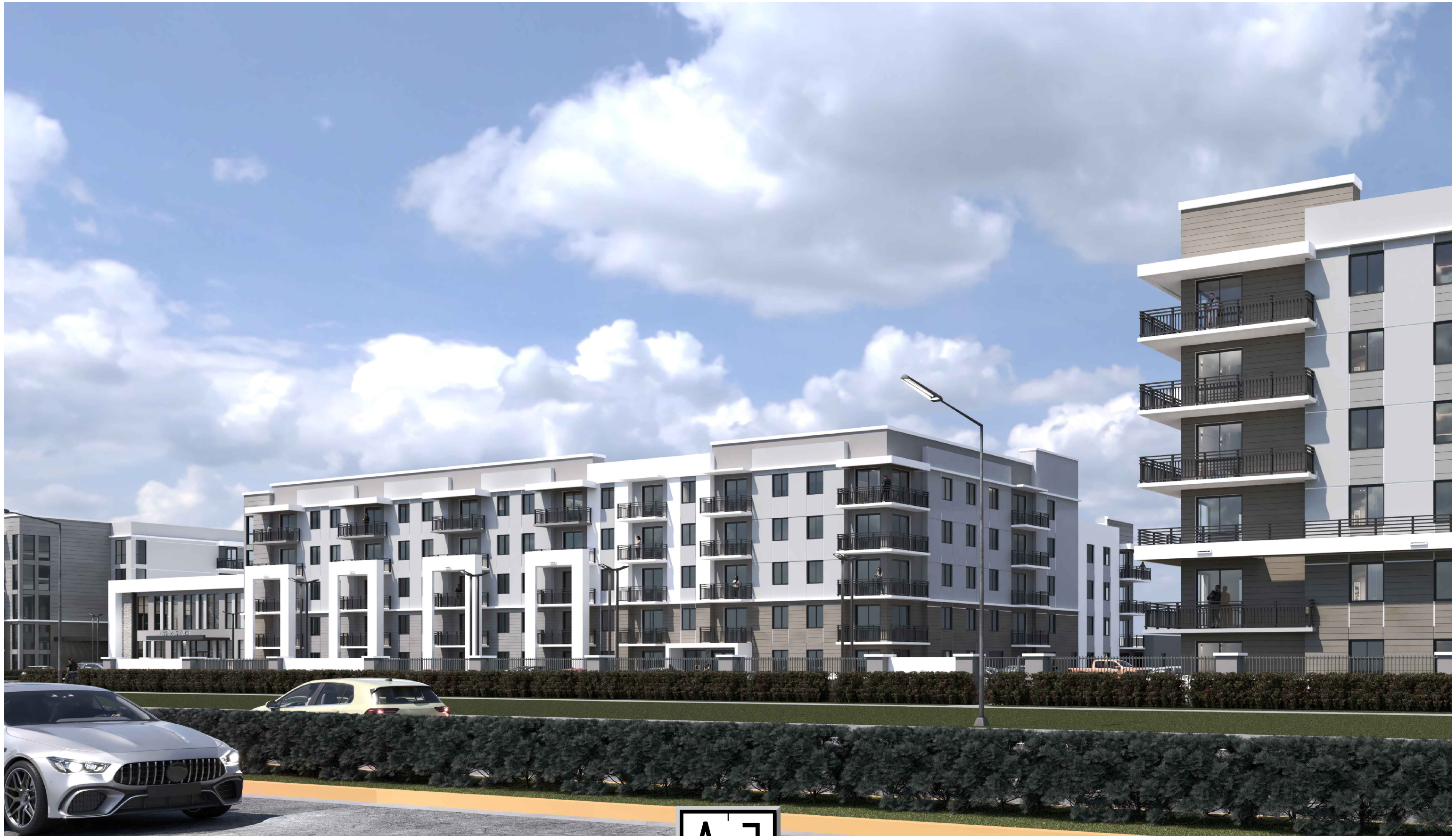
BLDG. 1 & BLDG. 2 NORTH SIDE (FROM W. OAKLAND PK. BLVD.)
