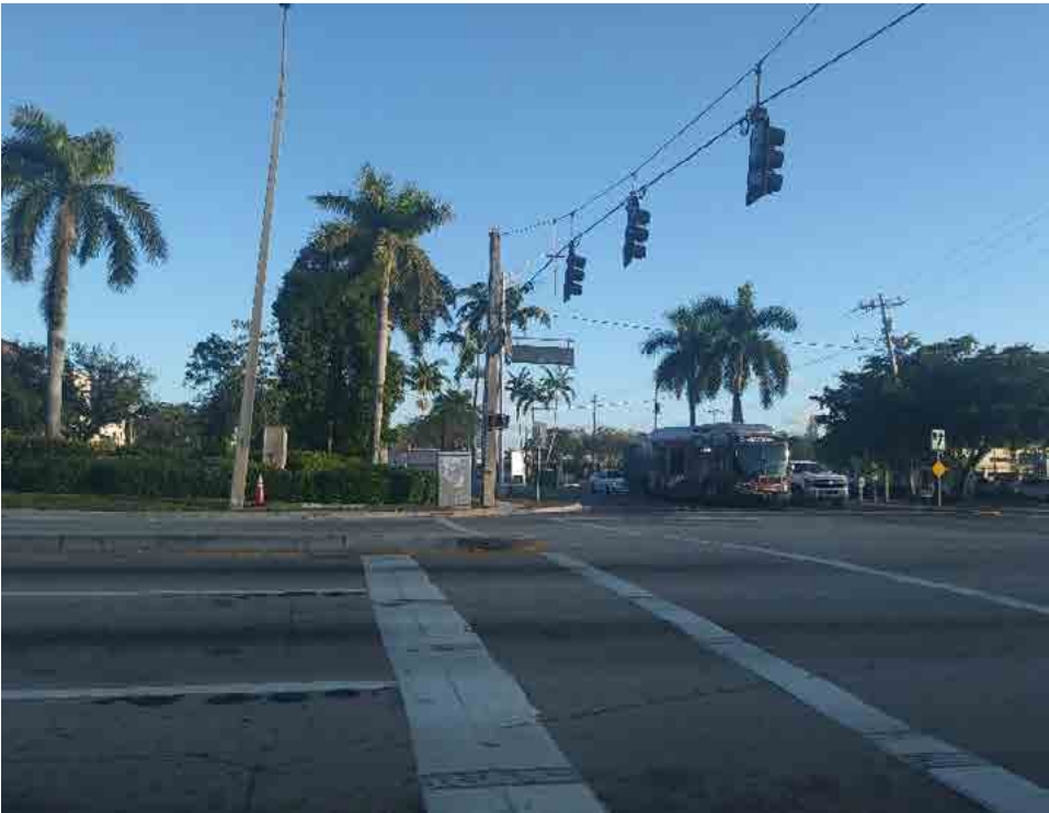
◀ Sunset Strip at Sunrise Boulevard existing crosswalk. Opportunity to improve crosswalk with textured/colored pavers
