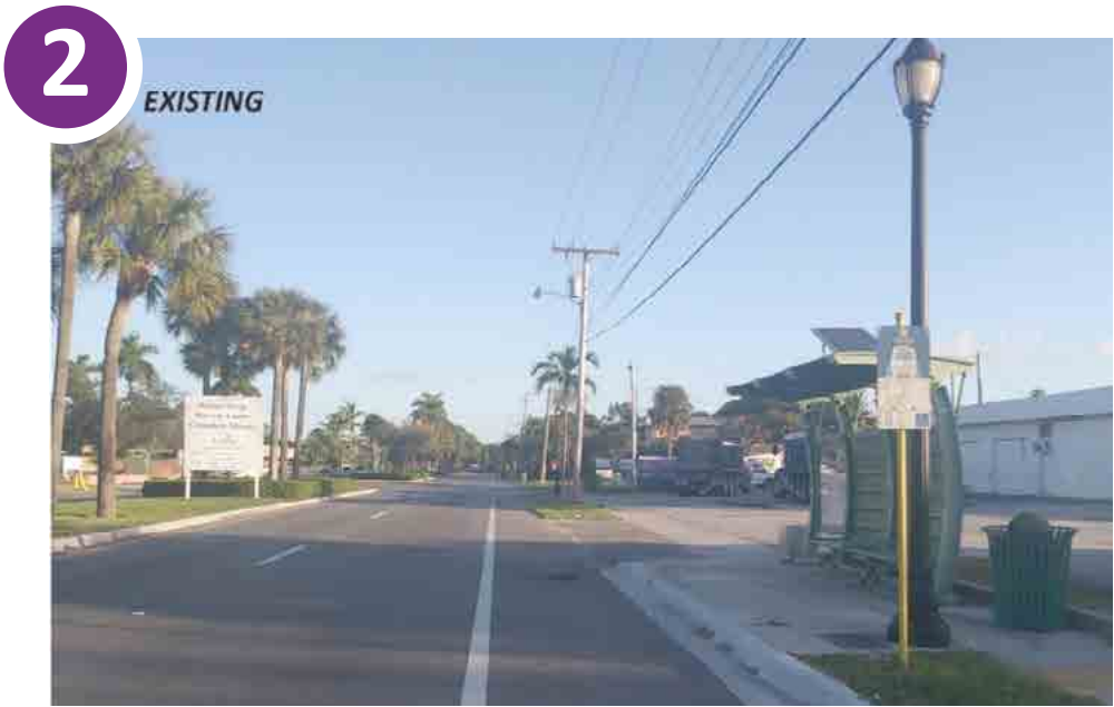
▲ Sunset Strip existing conditions
