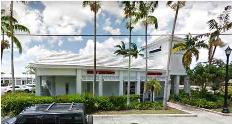
▲ Commercial with façade upgrades showcasing white architecture with tower, covered area, and slanted wood awnings.
